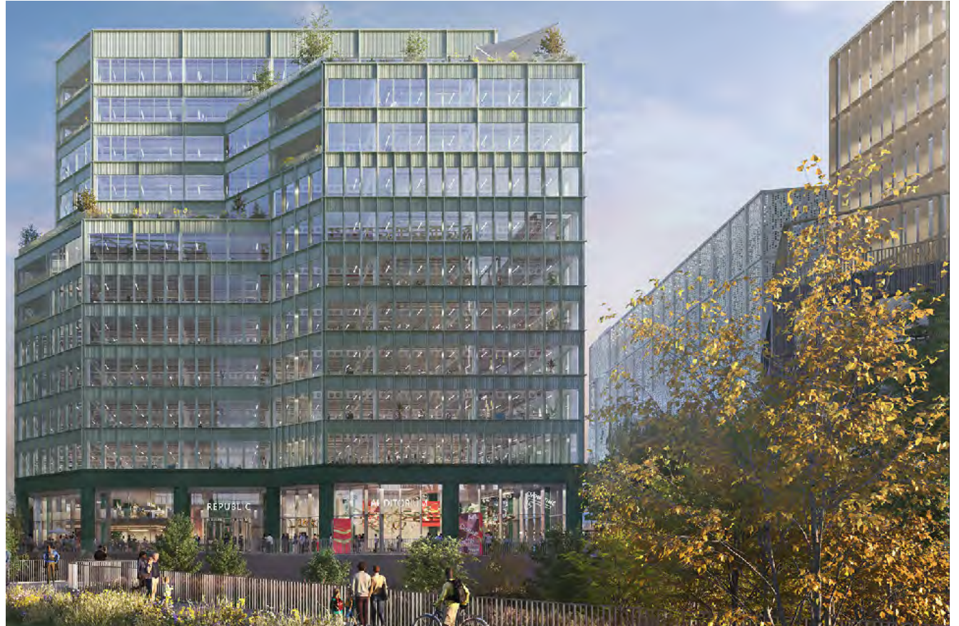
Baring Street Office 2 with the MSCP and Baring Street Office 1 to the right
